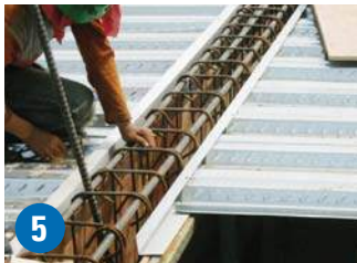
5 Fix steel edge form wherever required
