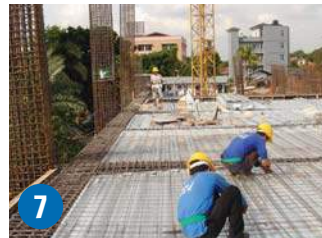
7 Place reinforcement
