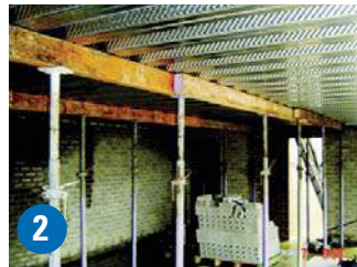
2 Place temporary support if required
