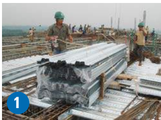
1 Place SMARTDEK™ sheet bundle on support
