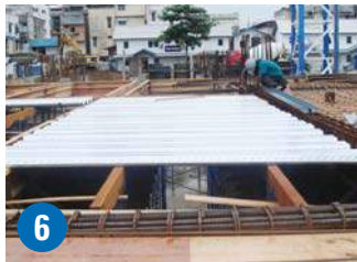
6 Fix SMARTDEK™ profiles to steel or concrete beam
