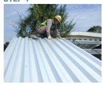
Place the second sheet with the female rib over-lapping the male rib of the first sheet. The sheets are snugly nested at the lap.
