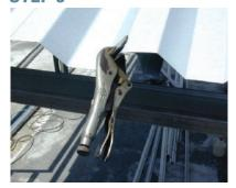
Vice grips are clamped on two ends. Fasten screws on the lap of every rib.
