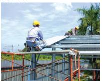
Locate the first roof sheet and make sure the female rib is close to the barge.
