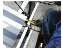
Check the end of roof sheet in relation to overhang for gutter.
