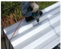
Fasten screws on each rib for single and end spans and every alternate rib for internal spans.
