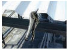
Vice grips are clamped on two ends. Fasten screws on the lap of every rib.
