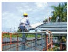
Locate the first roof sheet and make sure the female rib is close to the barge.
