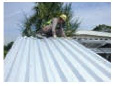
Place the second sheet with the female rib overlapping the male rib of the first sheet. The sheets are snugly nested at the lap.
