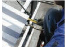
Check the end of roof sheet in relation to overhang for gutter.
