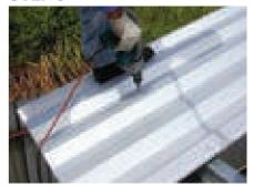
Fasten screws on each rib for single and end spans and every alternate rib for internal spans.
