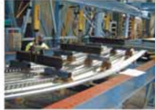
Formwork - Point Load
