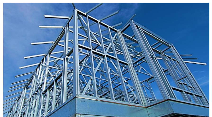
SMARTFRAME® light weight steel houseframing application
