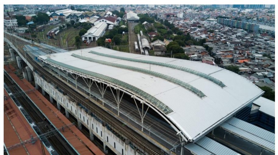
Manggarai Station is using LYSAGHT® FLEXLOK® COLORBOND® Gull Grey produced using Mobile Rollforming and On-Site Curving method.
