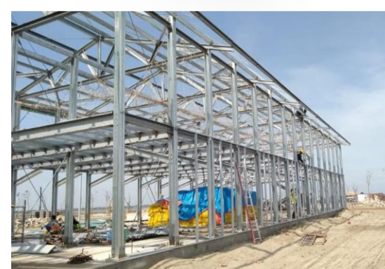
Patimban Port Office, Subang is using LYSAGHT® Cee Purlins as main structure for Pre-Engineered Building System
