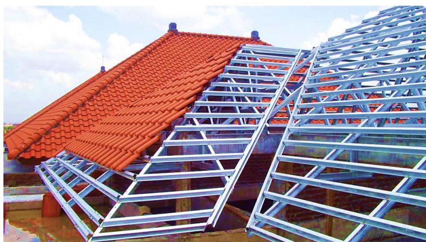
SMARTRUSS® light weight steel roof truss application
