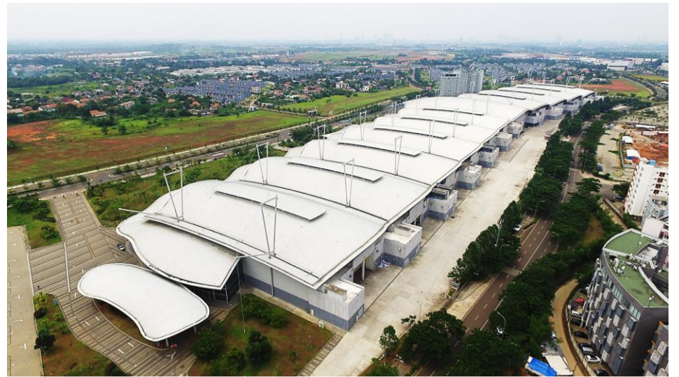
ICE BSD is using LYSAGHT® FLEXLOK® COLORBOND® Gull Grey produced using Mobile Rollforming and On-Site Curving method.
