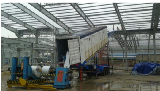
Mobile Elevated Rollforming (MERF)
