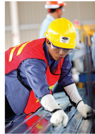
Can be fabricated off-site and delivered pre-assembled
