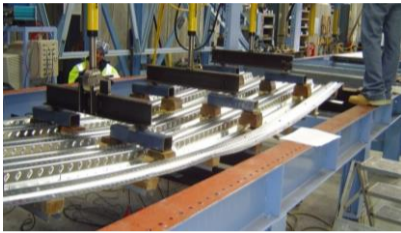
Formwork – Point Load
