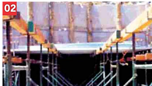
2 Place temporary support if required
